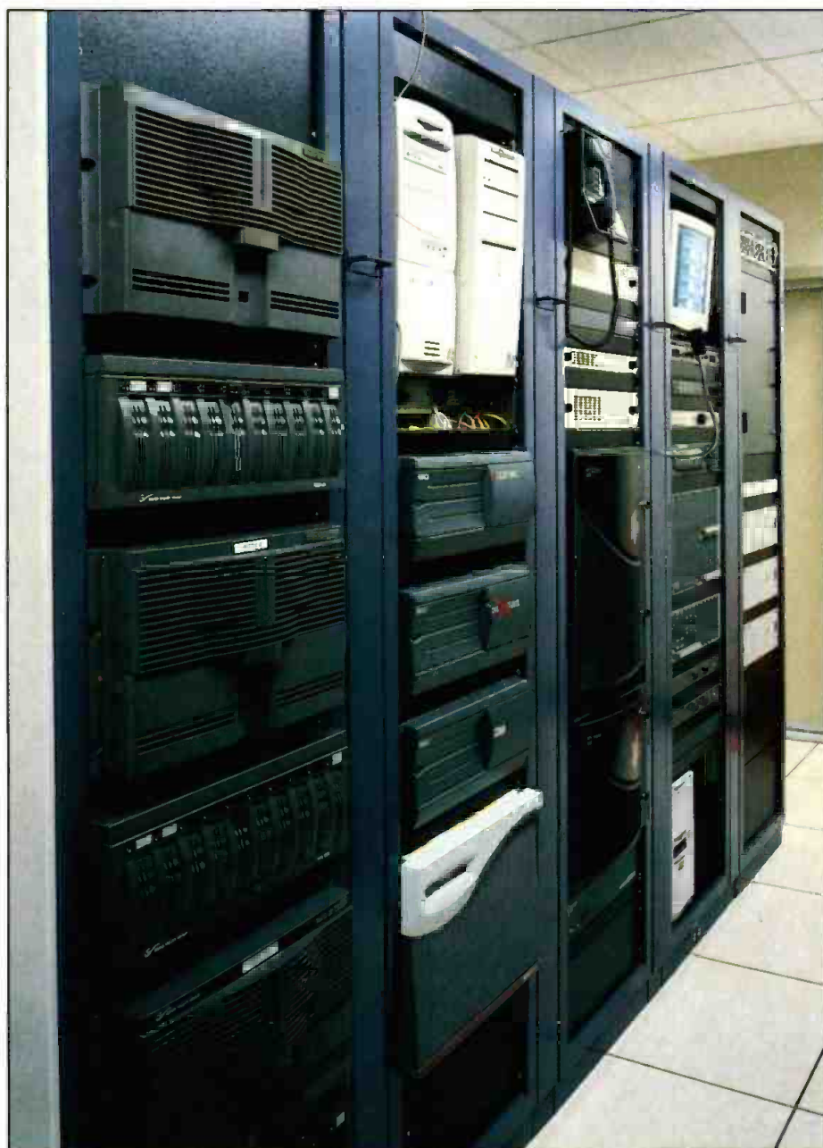
Shown above is a set of racks in KPDX's main technical core, containing the Profile XP server system, the Pinnacle and Quantel graphics mainframes, the main router, intercom and digital camera base stations.
