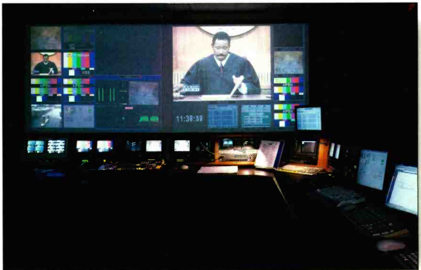
The design team incorporated a 16' x 7' projection screen (shown above) into master control, displaying output from two Miranda Kaleido multi-image processors. Images from up to 32 separate sources at one time can be shown on the wall.
